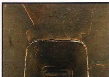
Actual photo of cracked flue tiles
